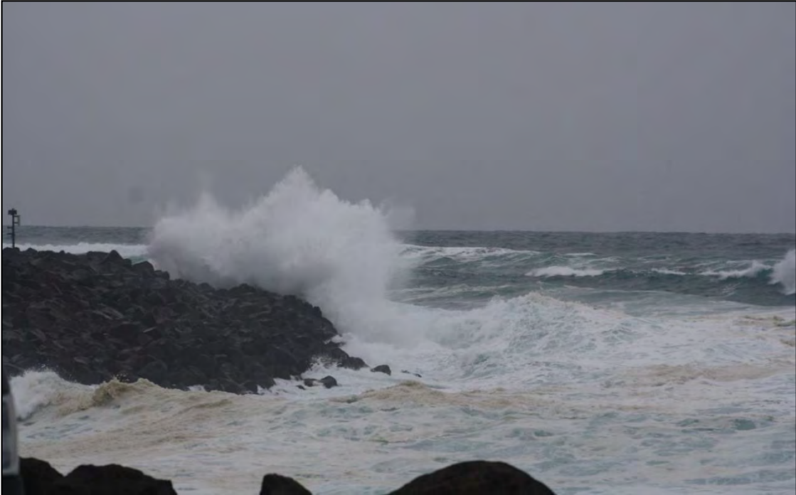
Figure 11. St. George Harbor South Breakwater, February 13, 2018, Southwesterly Storm.
